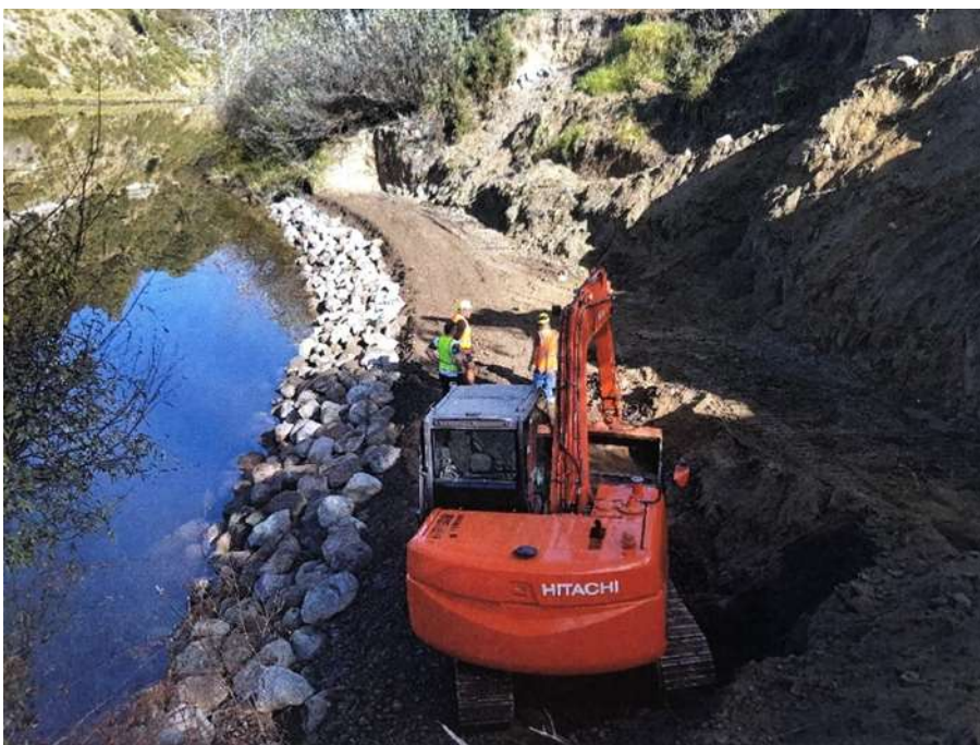
Photo: Rock lining being completed on lower river bank, Jerusalem
